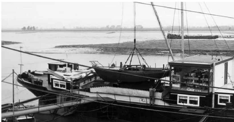
M Engelaer Shipbuilding around 1965. After the aft sections of two large tow barges were welded together, one work space and two living quarters were created. In the derrick hangs the steel hull of a Gouwzee cruiser the Engelaers built for Pieter Beeldsnijder.
